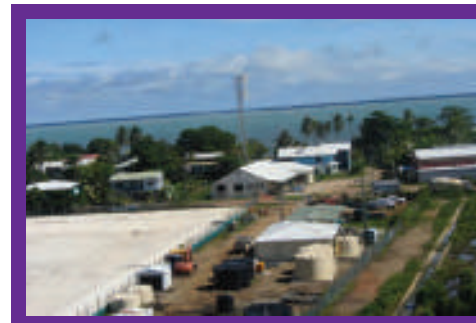
INDUSTRIAL - SHEDS / WORKSHOP / LAYDOWN
