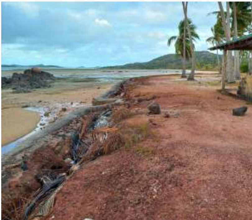
Seawall at Badu
